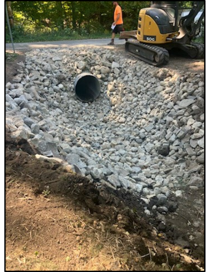
ACRES Land Trust Ball Lake Easement during grade stabilization construction Photo courtesy of Kent Tracey, NRCS Engineering Technician
